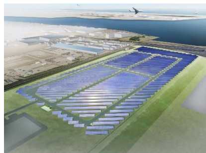
Solar power plant
