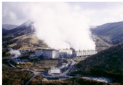
Geothermal power plant
