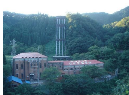
Hydroelectric power plant
